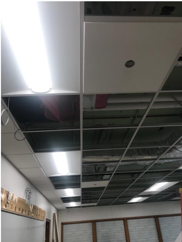
Installed Light Fixtures
