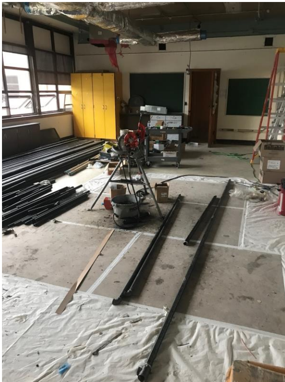
Sprinkler Pipe Fabrication
